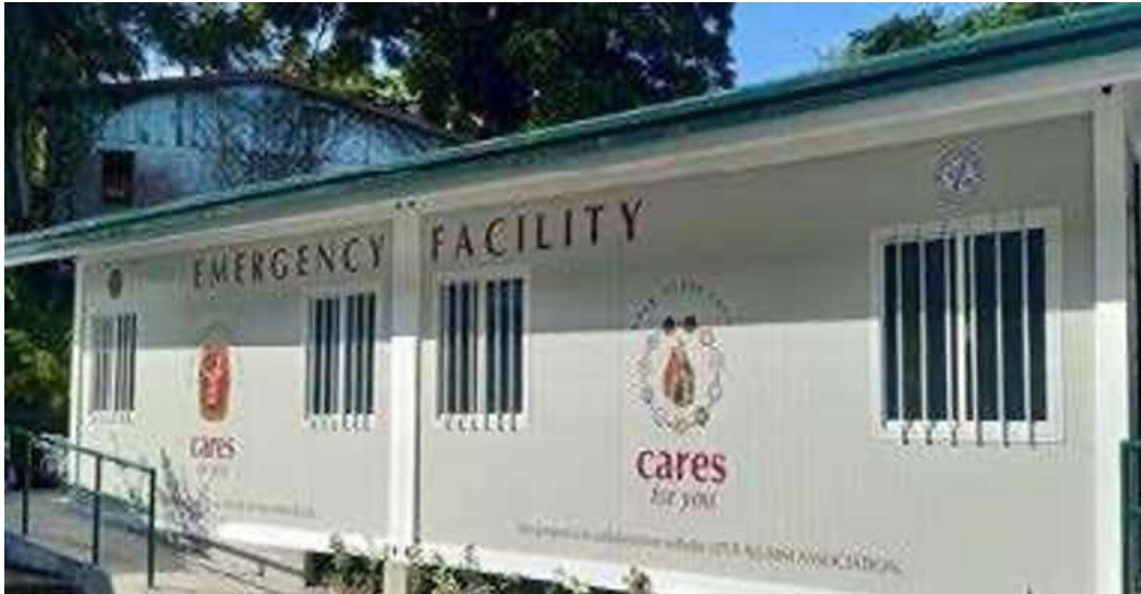
UHS Emergency Room Extension Facility
