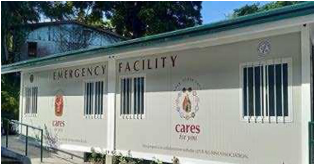
UHS Emergency Room Extension Facility
